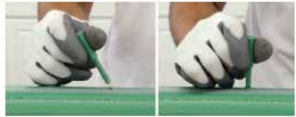
Picture no. 48: Inserting the repacking plug
