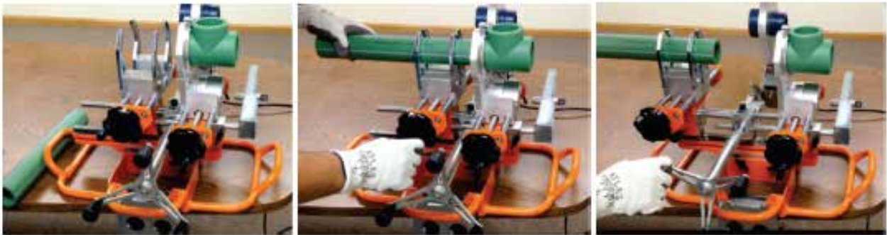
Picture no. 37: Pipe and fitting alignment procedure
