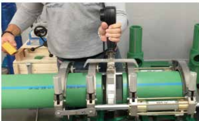
Picture no. 43: Insertion of the heating plate
