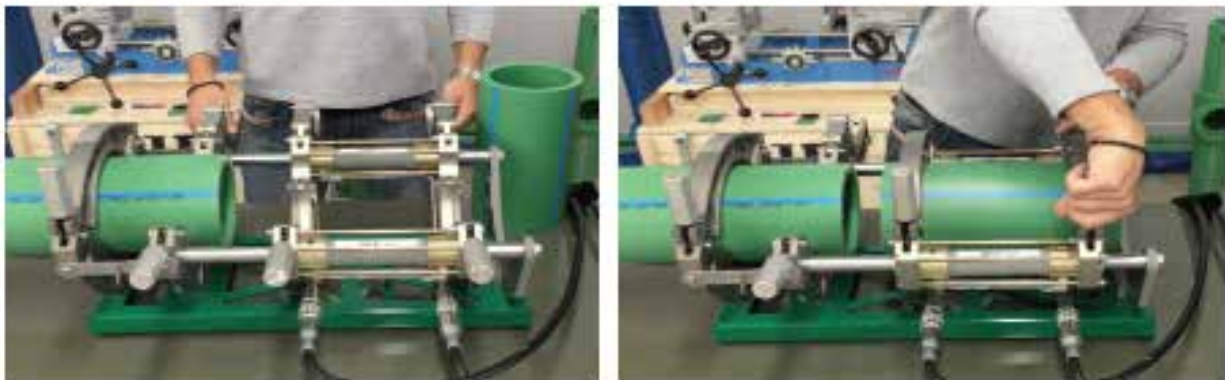
Picture no. 41: Fixing the pipe with jaws
