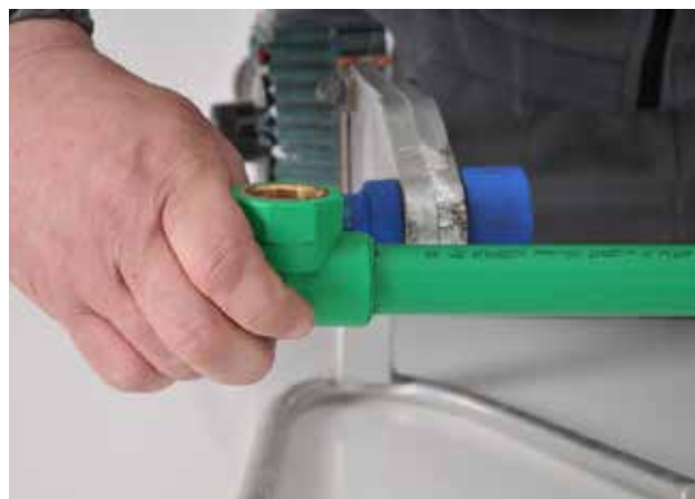
Picture no. 25: Connecting pipes and fittings
