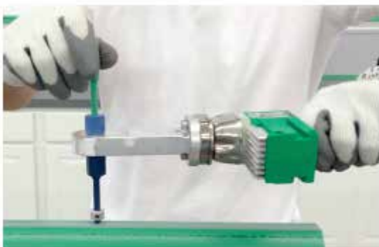
Picture no. 47: Inserting reparation tools
