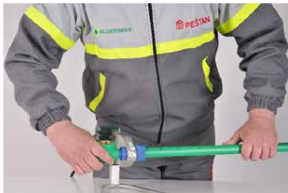
Picture no. 23: Heat pipe and fittings (pay attention to positioning the pipes and fittings on the heating plate)
