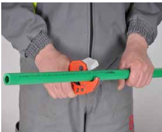
Picture no. 19: Cutting PP-R and PP-RCT pipes
