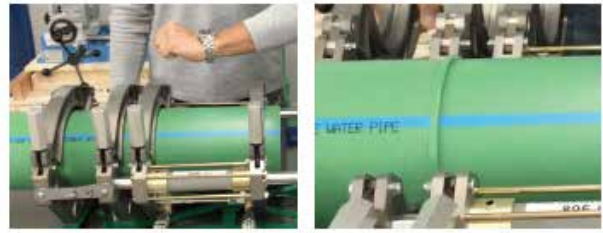
Picture no. 44: Butt Welding
