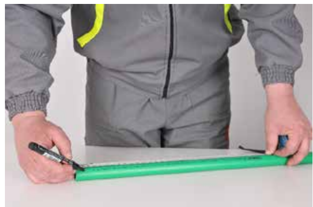
Picture no. 21: Marking the required depth of cheeses. The required welding depths along pipe diameters can be taken from the following table:
