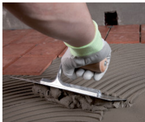
Application of Granirapid on terrace waterproofed with Mapelastic Zero
