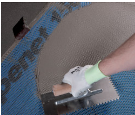
Application of Mapelastic Zero on Mapenet 150
