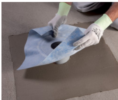
Application of Drain Vertical on Mapelastic Zero
