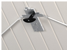
Lock with a lock cylinder bolting the door on both sides
